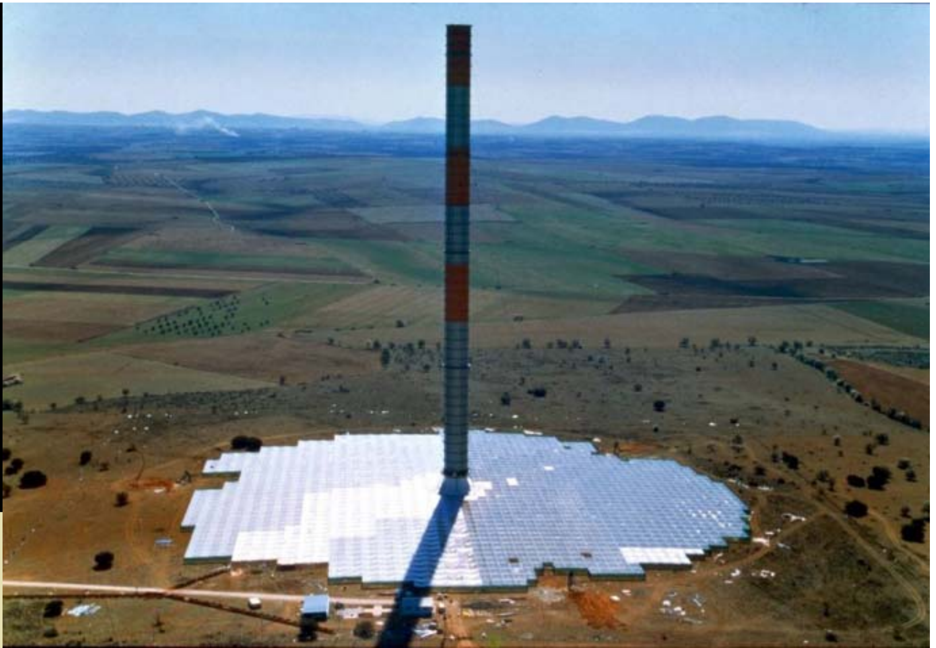
Solar Chimney Manzanares, Experimental Plant 1982, Spain
